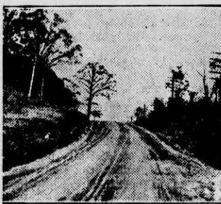
Good Road Crown Maintained by Draining in Alexandria County, Virginia.
